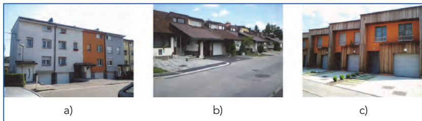
Figure 24.2. Attached houses: a) 1960-70s; b) 1980-90s; c) after 2000.
