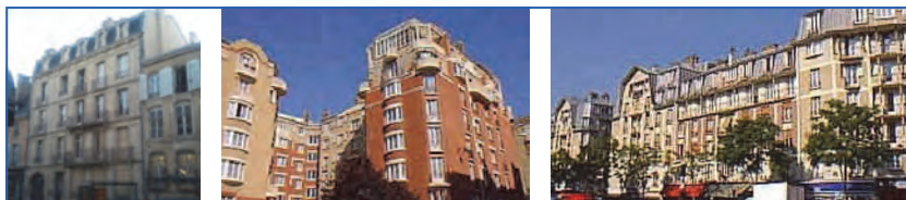
Figure 8.14. Example of buildings between 1914 and 1948 (from [2] and www.parisbalades.com ).
