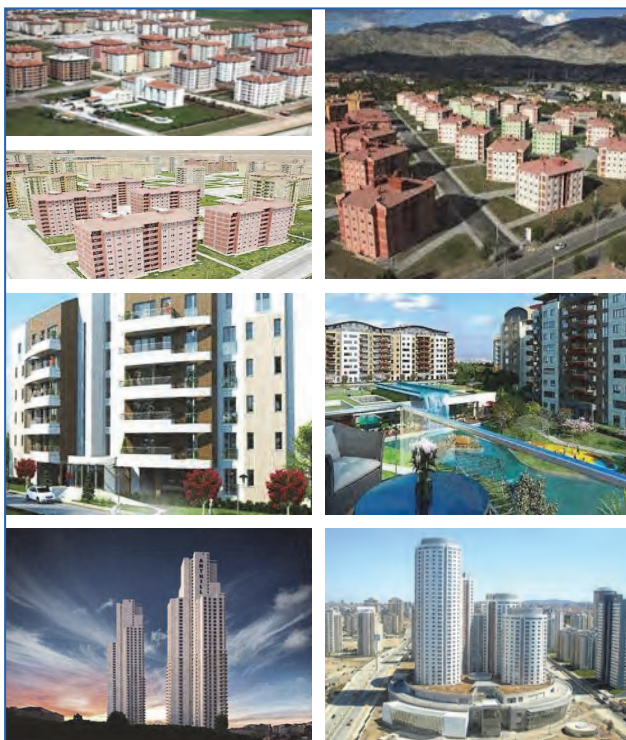
Figure 28.6. Samples of the building sites. First row (1,2): Mass houses built by Government (TOKI) especially in earthquake regions and urban transformation areas (concrete frame and all walls of gas concrete). Second row (3,4): New suburban neighbourhoods (buildings with concrete frame and gas concrete walls, some gypsum board interior walls). Third row (5,6): High-rise residential blocks in Istanbul (curtain walls, some steel framed, interior walls of gypsum board constructions). Ref. [4].
