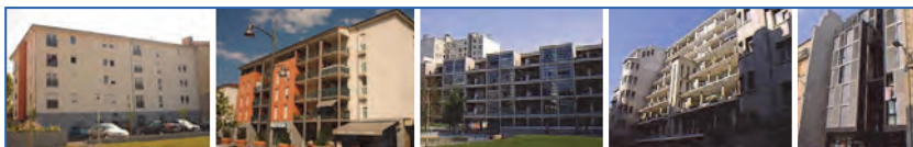
Figure 8.19. Example of buildings between 1990 and 2000 (from [2] and www.parisbalades.com ).
