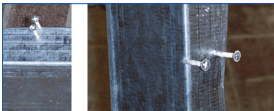
Figure 1.15. Position of the screws: left optimal, right suboptimal.
