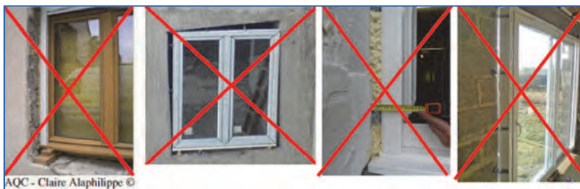
Figure 8.10. Example of problems related to windows.
