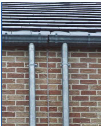
Figure 2.37. The interruption of the outer façade wall will allow gaining 1 or 2 dB extra in sound insulation.
