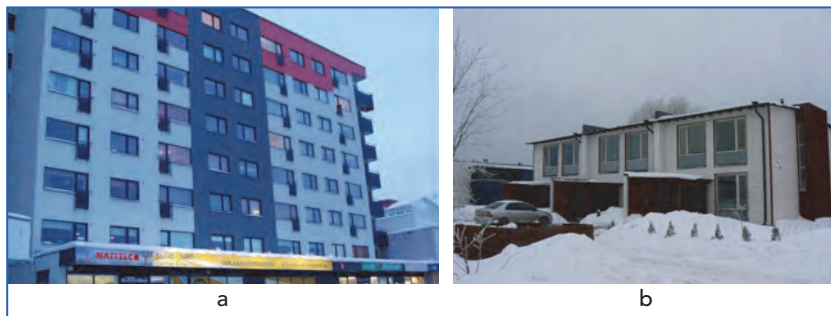
Figure 6.4. Photos: a) Massive structures a; b) Detached row-house.
