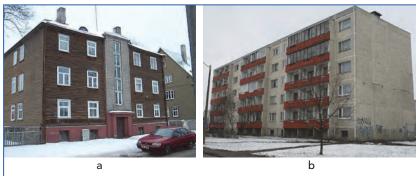
Figure 6.8. Photos: a) Wooden building; b) Concrete element building.
