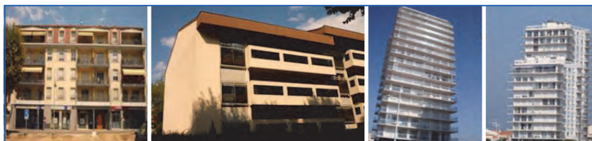
Figure 8.17. Example of buildings between 1974 and 1981 (from [2]).
