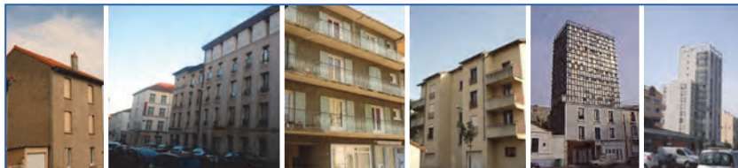
Figure 8.16. Example of buildings between 1968 and 1974 (from [2] and www.parisbalades.com ).
