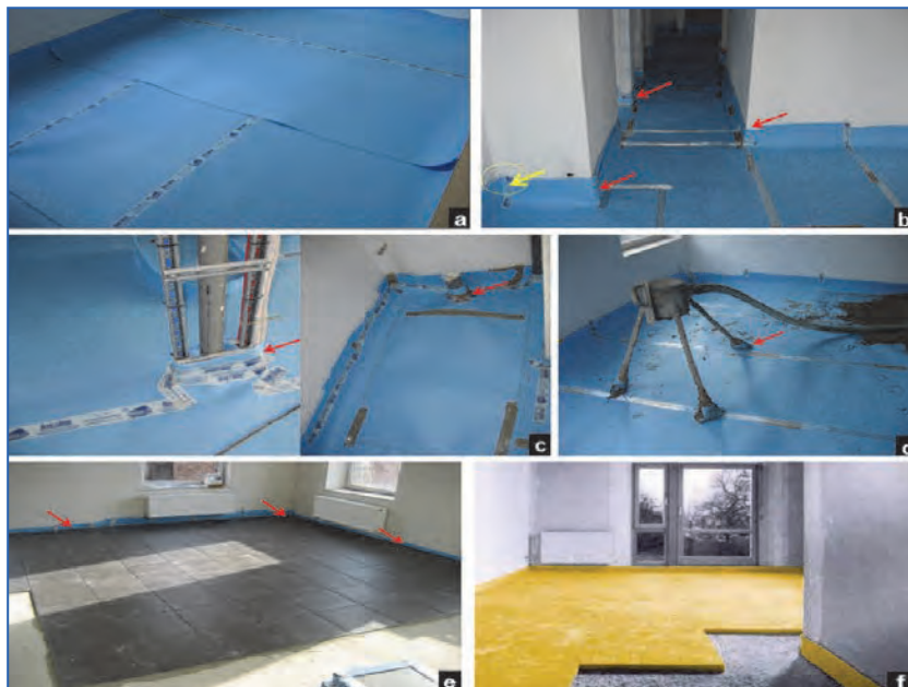
Figure 2.35. Correct mounting of a floating floor.
