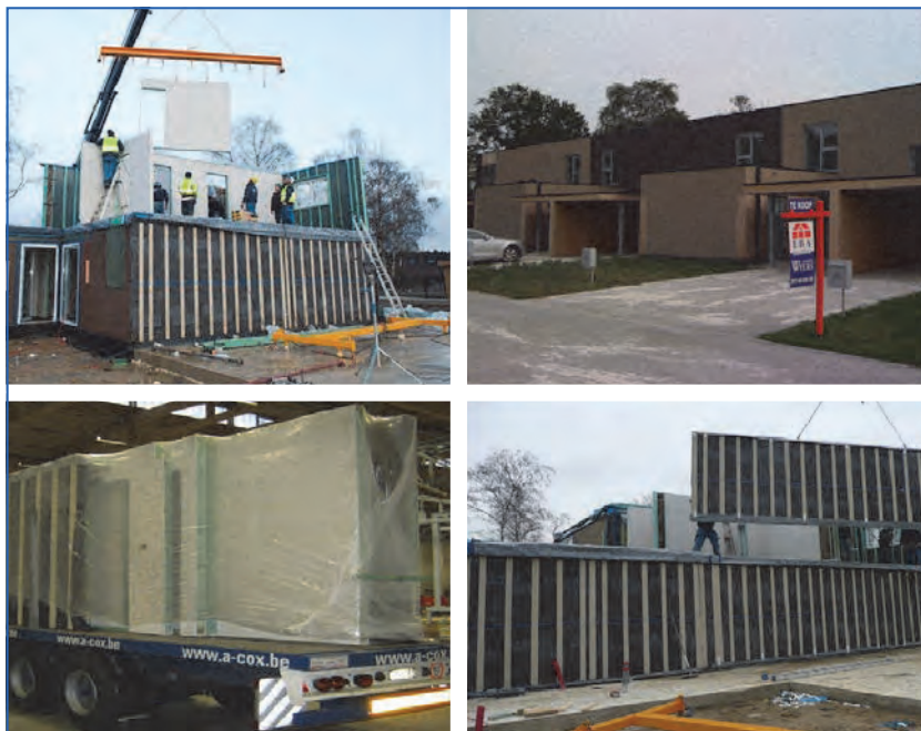
Figure 2.24. The newly developed party wall with improved fire and acoustic performances, are now regularly being built (prefabrication).
