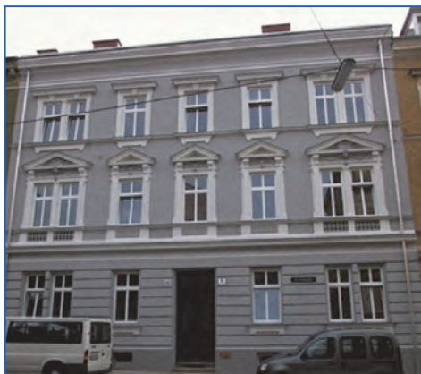
Figure 1.29. Example of a residential building in Linz (capital of the province of Upper Austria), built during the first half of the 20 th century, brickwork walls and timber floors.
