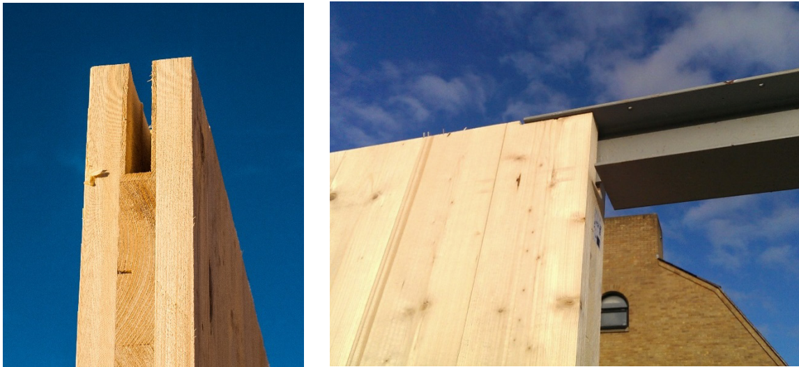
Fig. 17 Special detail to support end bearing of a steel lintel beam.
