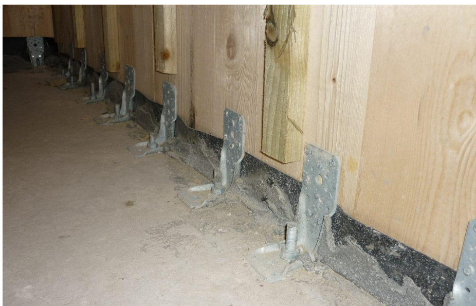
Fig. 9 Typical CLT wall to concrete connection with grouted gap at wall base.
