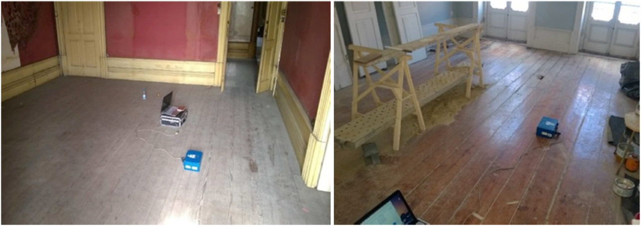
Figure 5: Dynamic identification of timber floors (with floorboards)
